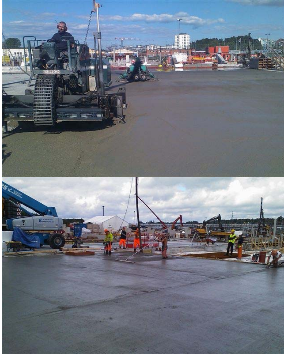
Fig.7 Laser screeder and hand laying of the slab
