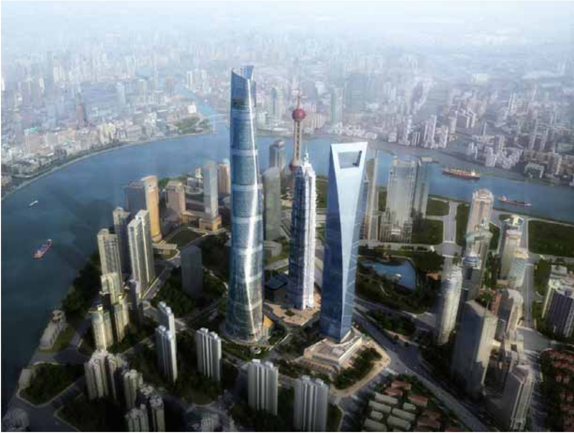
Shanghai Tower 632 m
