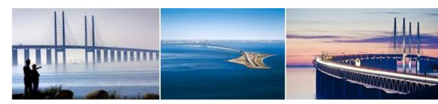
The Öresund Bridge is a double-track railway and motorway bridge across the Öresund strait between Sweden and Denmark. The bridge runs nearly 8 kilometres from the Swedish coast to the artificial island of Peberholm, which lies in the middle of the strait. The crossing of the strait is completed by a 4 kilometres underwater tunnel, called the Drogden Tunnel, from Peberholm to the Danish island of Amager.
