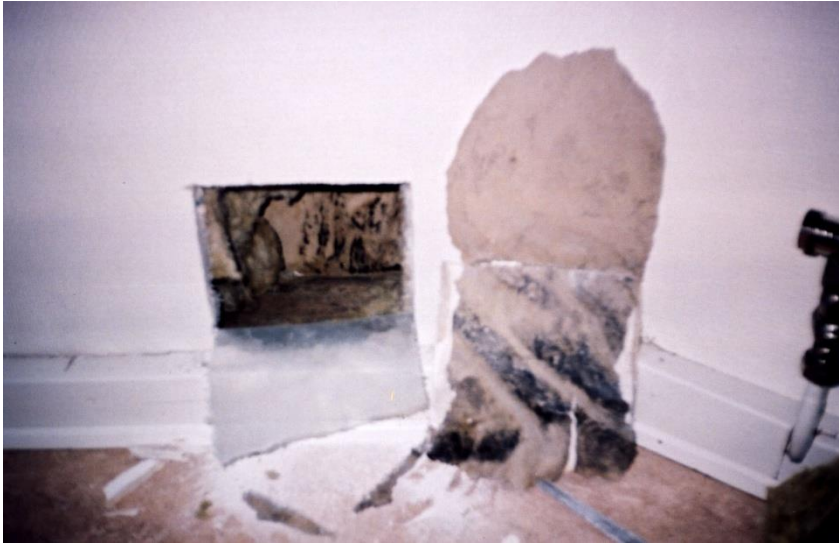
Typical Swedish moisture damage
