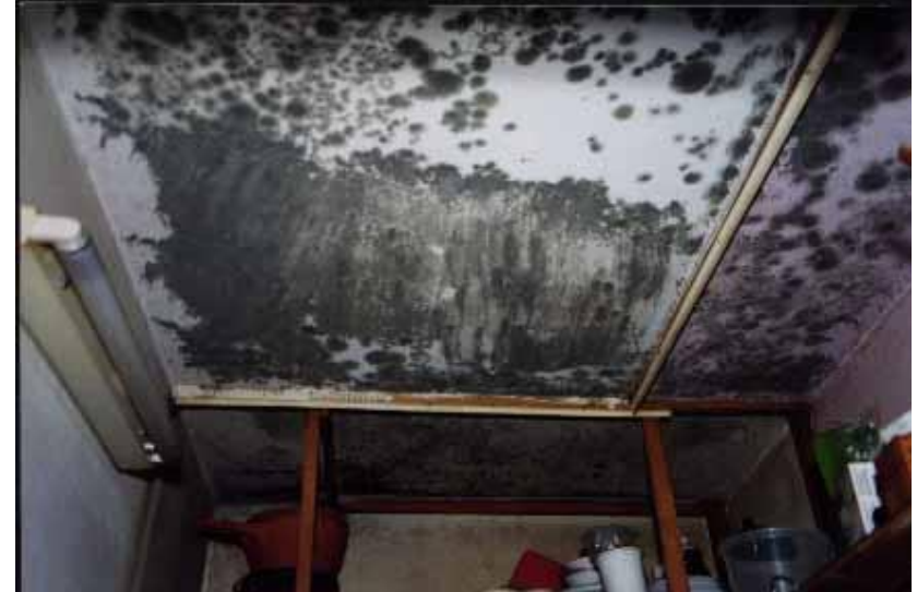
Mould on internal surface, unusual in Sweden
